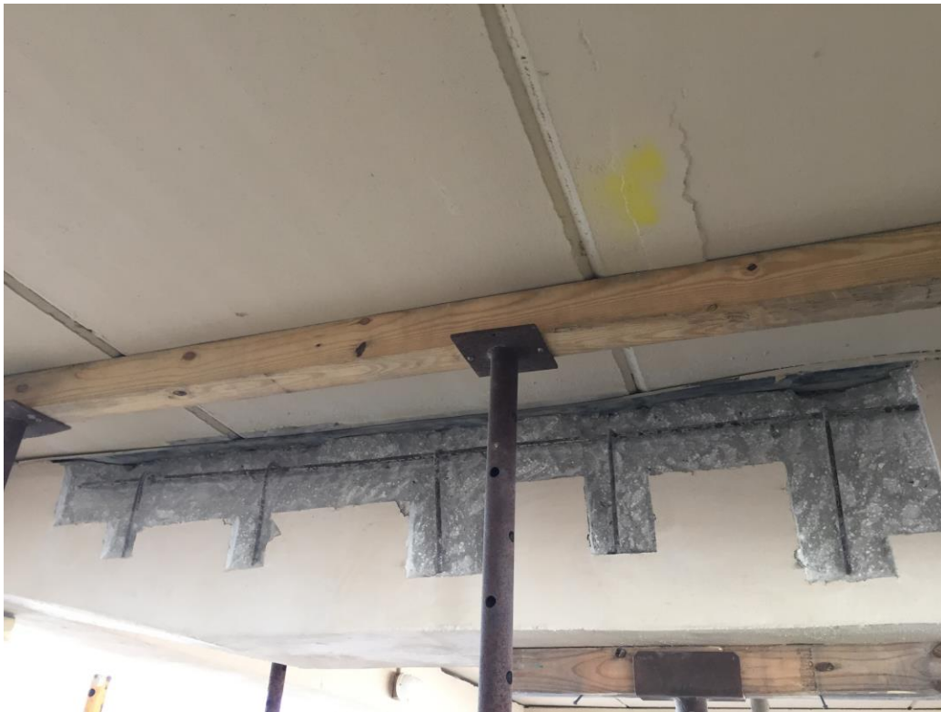
Picture 4: In-progress concrete repairs
