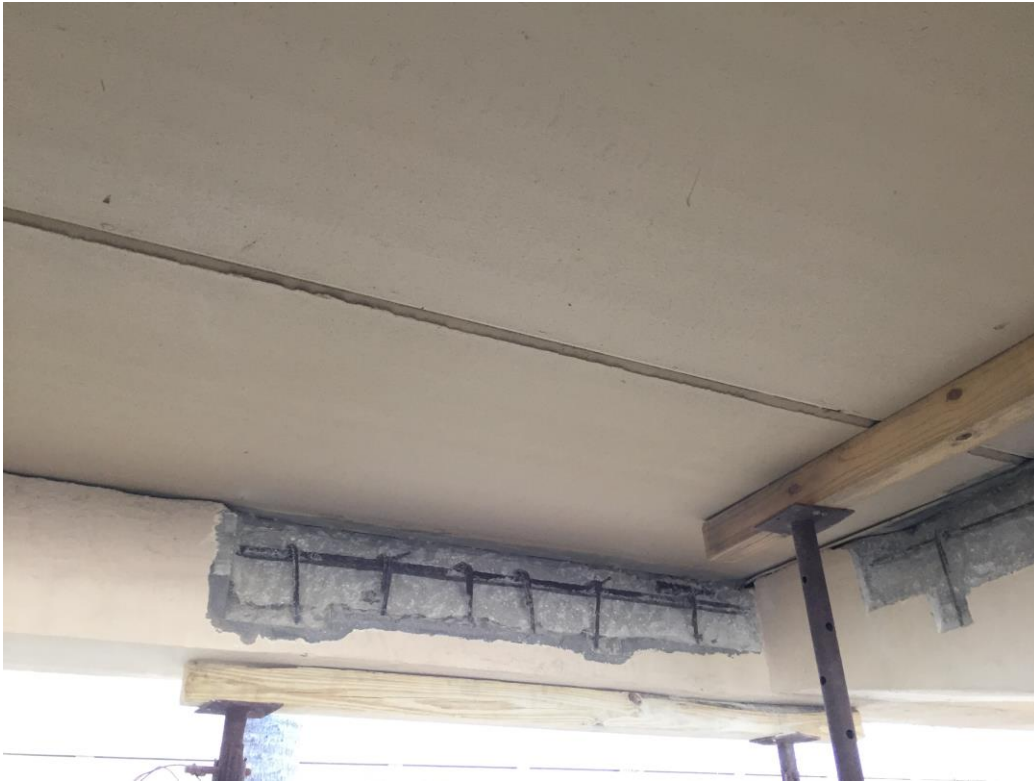
Picture 3: In-progress concrete repairs
