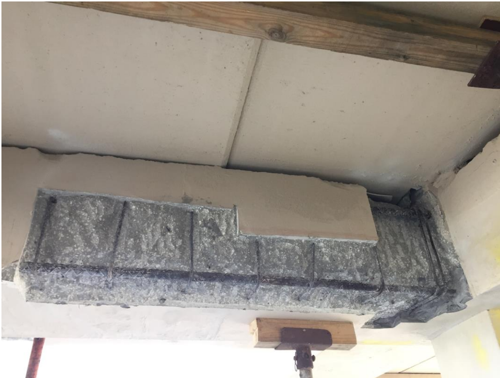
Picture 2: In-progress concrete repairs
