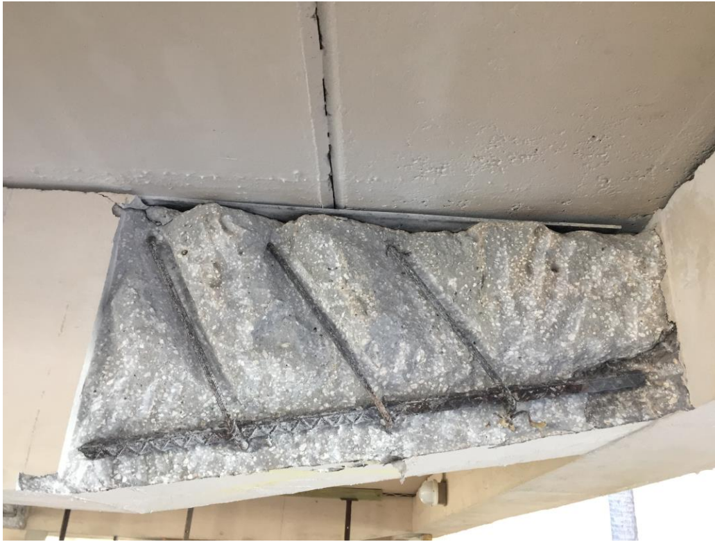
Picture 1: In-progress concrete repairs
